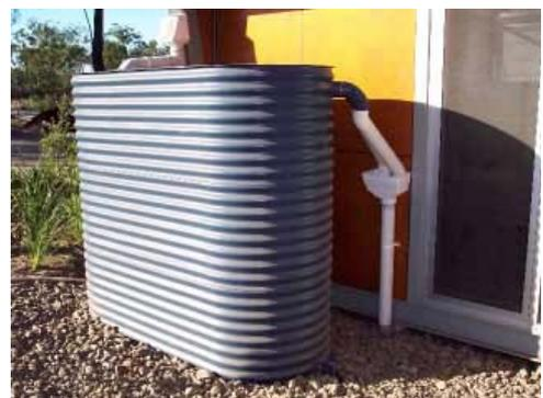
Once it is known how much water can be collected and how much water is going to be used, then a tank size can be selected that will ensure the reliability of water supply that is needed.
