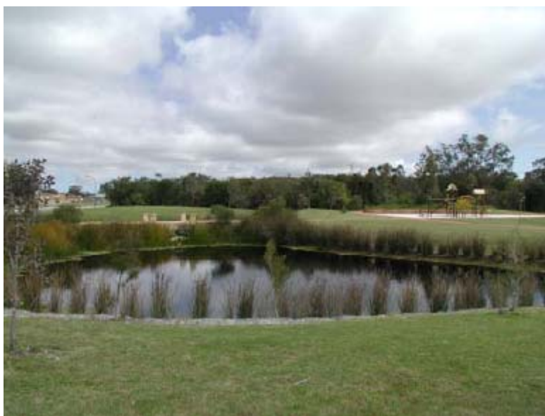
Figure 9.12 Sediment Settling Basin in Perth, WA
