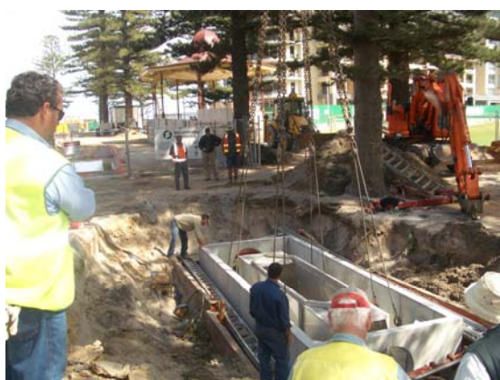
Figure 9.15 Augusta Street, Glenelg - GPT Installation
