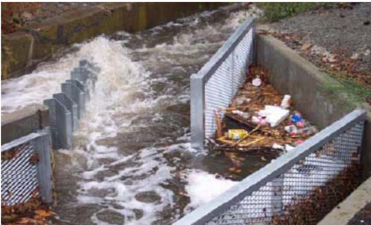
Figure 9.9 Vane Style Diversion Weir, Sebastopol, Victoria
