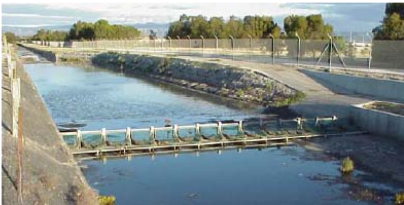
Figure 9.7 Channel Nets at West Torrens, Adelaide, SA
