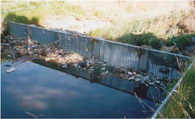
Figure 9.8 Trash Rack Installed at Broadmeadows, Victoria
