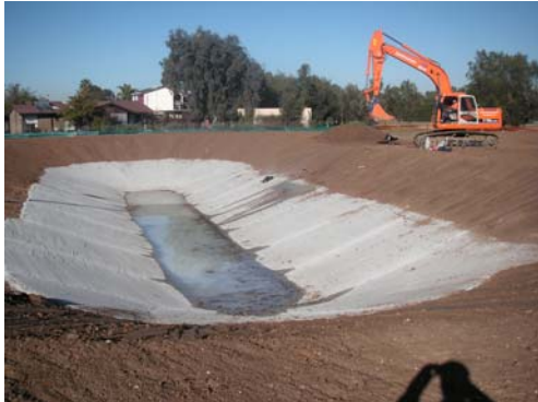
Figure 8.4 Grange Golf Club Stormwater Harvesting and Reuse Scheme - During Construction (June 2006)
