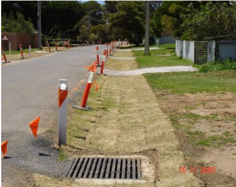
Figure 11.1 Palmer Street Swale Retrofit, Aldinga Beach
