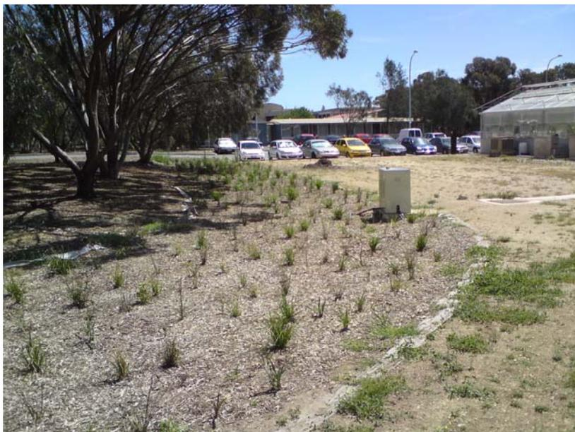
**Figure 1.2** Bioretention Swale, Mawson Lakes, SA
