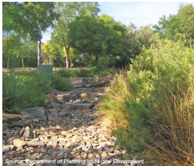
Condition of the detention swale in February 2010
