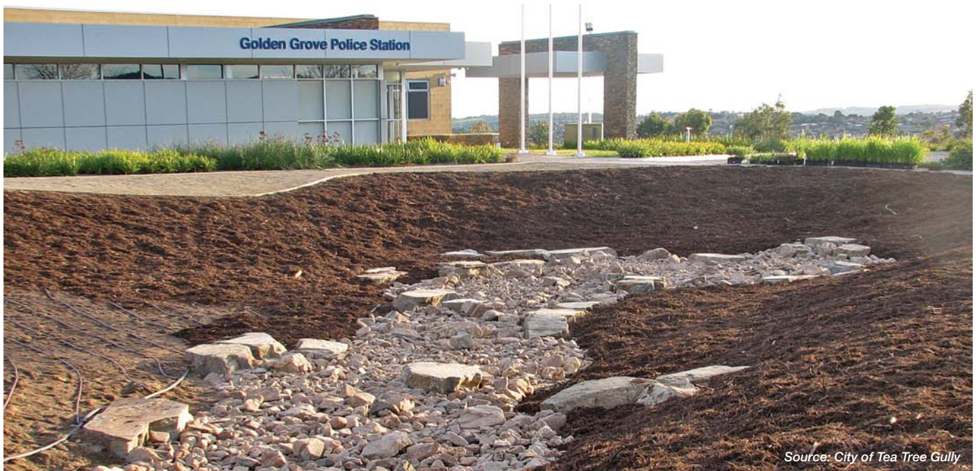
Completed swale and rock lining (looking towards sump)
