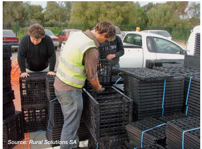
Construction phase: assembling crates for the sump
