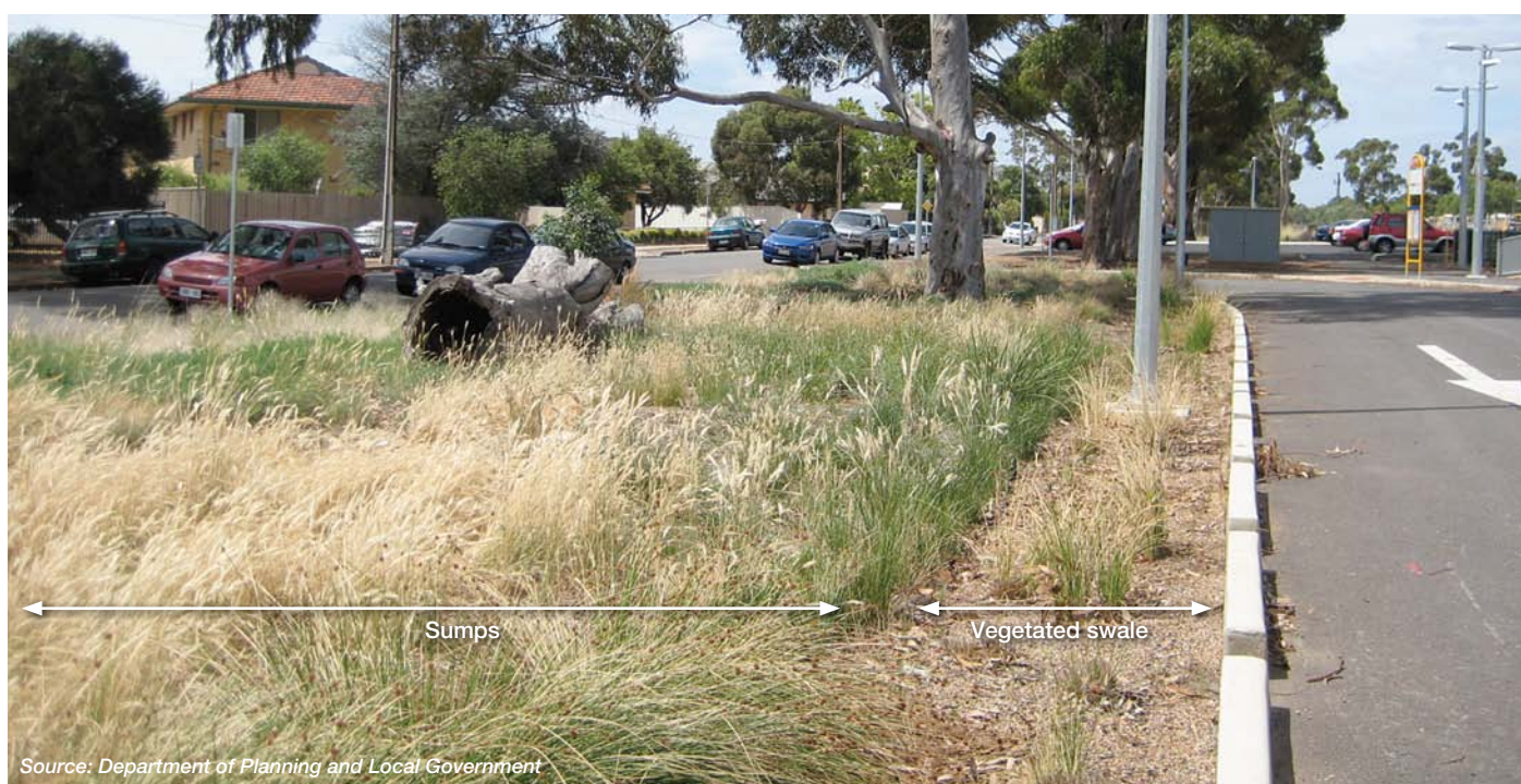
Ficinia nodosa and Austrodanthonia spp. growing well in the natural soil on the sump (left), while some of the Ficinia nodosa plants in the swale (right) are drying out
