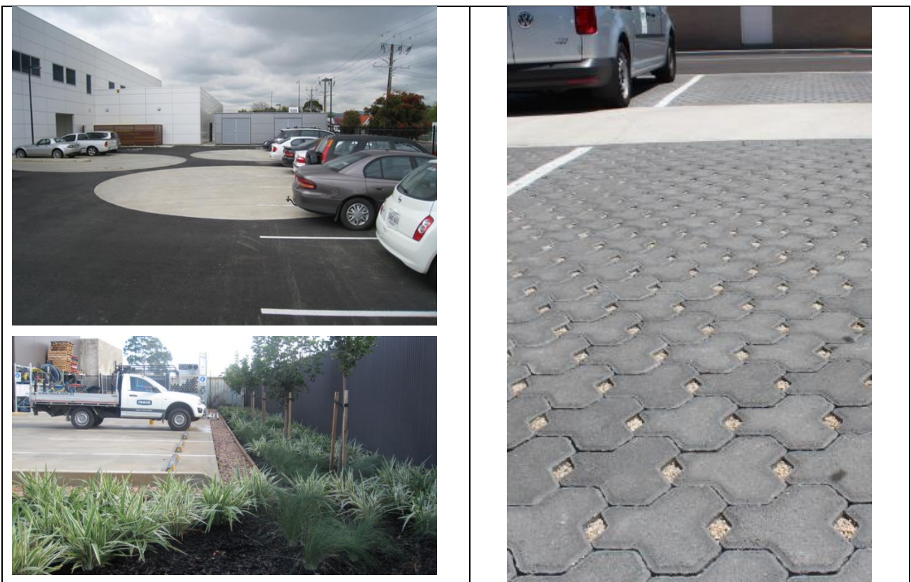
Figure 1: Clockwise from top left – underground rainwater storage tanks (one detention and two retention tanks), permeable paving, raingardens (Source: Andrew King)
