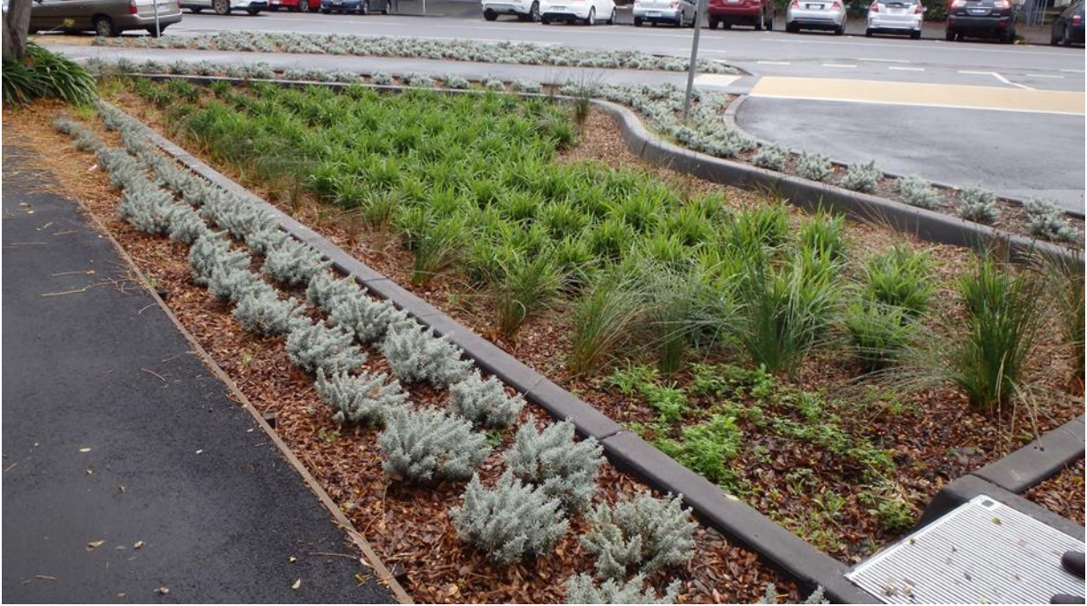
Figure 6.8 Streetscape bioretention, South Melbourne (E2Designlab, 2014)
