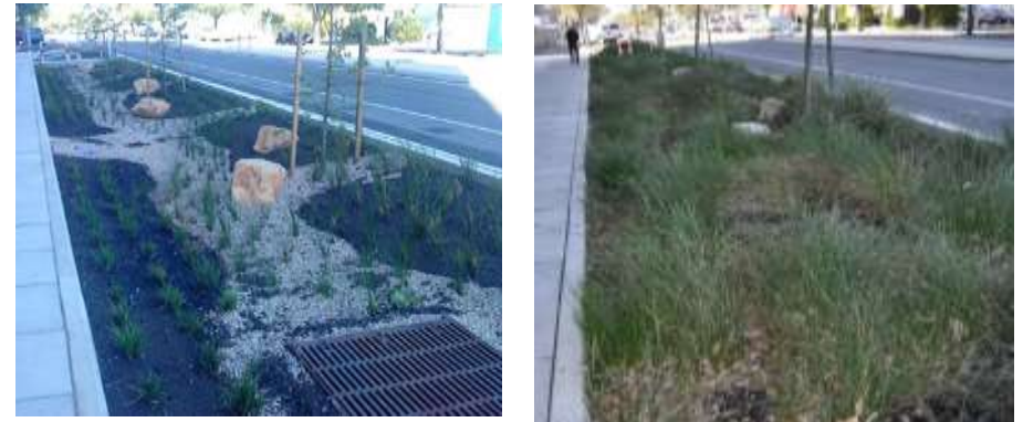
Angas Street, Adelaide raingarden (i) showing arrangement of filter media and (ii) once established.
