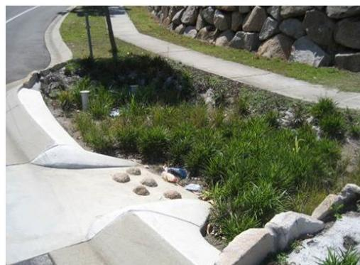
ight) at the **inlet** to a biofilter can be used reduce flow our and erosion damage.
