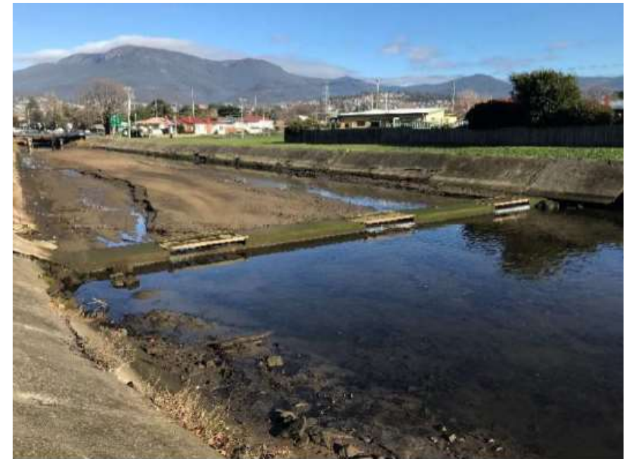
Weir and view upstream towards Queens Walk
