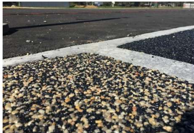
Figure 10: Laura Avenue, St Marys porous asphalt surface in the , City of Mitcham and Cowandilla Community Hall carpark, City of West Torrens
