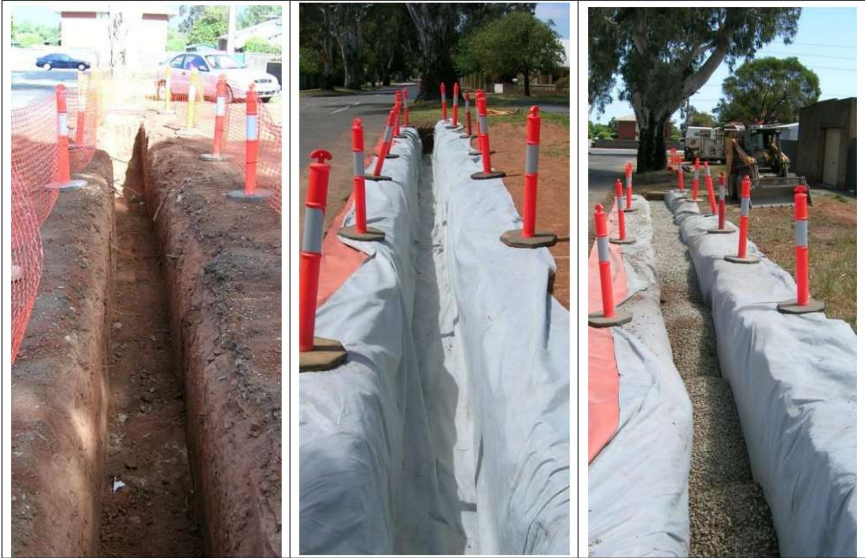
Figure 9: Infiltration trench, Doncaster Avenue, Colonel Light Gardens, City of Mitcham
