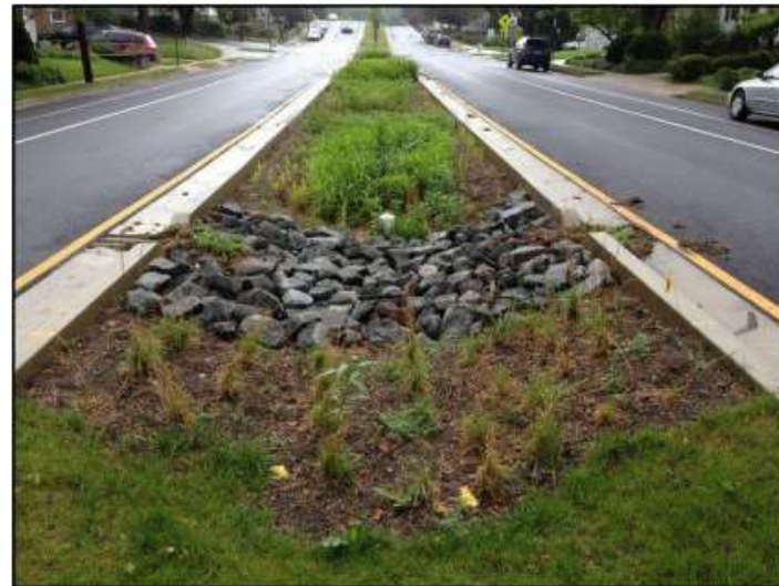
Figure 13: Typical raingarden barrel/tank (top left), bioretention basin/raingarden (top right) and bioretention swale (bottom) installations
