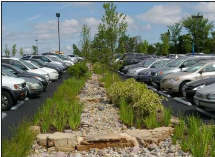
Figure 13: Typical raingarden barrel/tank (top left), bioretention basin/raingarden (top right) and bioretention swale (bottom) installations
