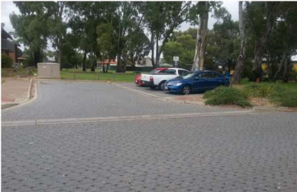
Figure 12: Permeable paving Kegworth Road, Melrose Park, City of Mitcham
