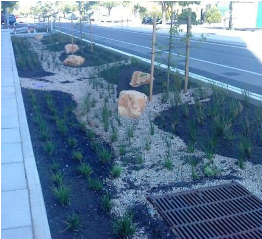
Angas Street raingarden early and established, showing arrangement of filter media
