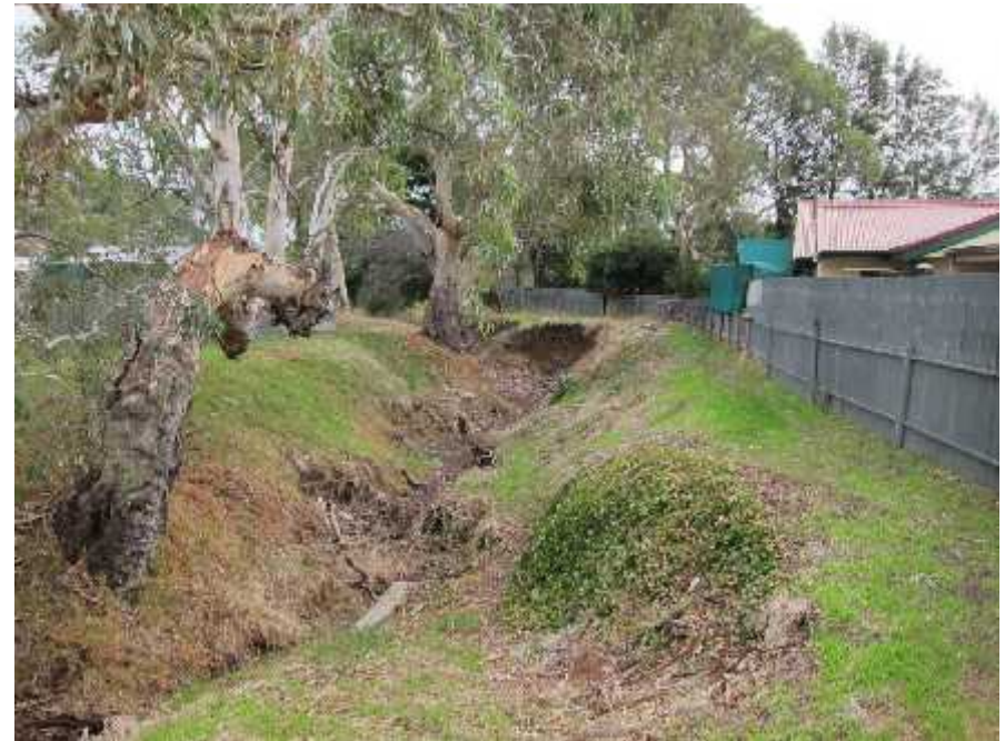
Thrushgrove Creek, City of Onkaparinga. Note erosion of banks due to frequent high flows. These destructive flows are caused by urbanisation.
